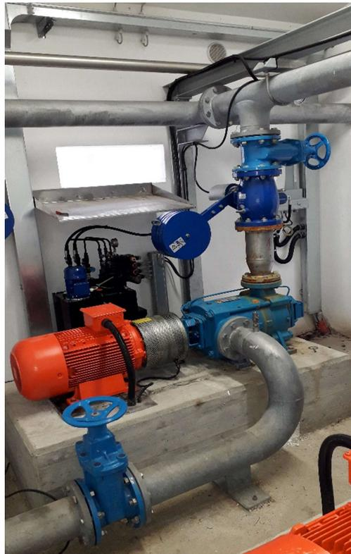
Figure 1 – Pelton turbine installed in micro-hydropower station
