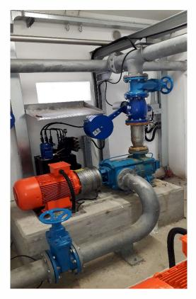
Figure 1 – Pelton turbine installed in micro-hydropower station
